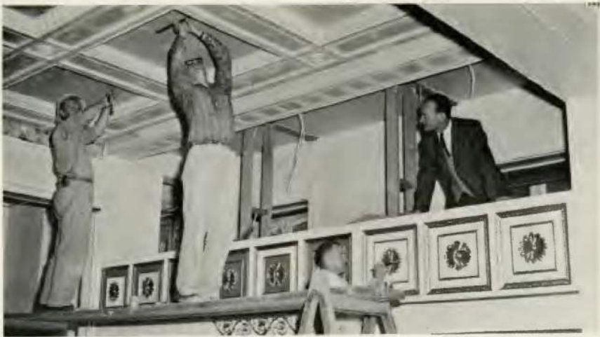
Fixing the components of the Adam coffered ceiling
